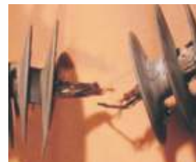
Cracks in Polymer
