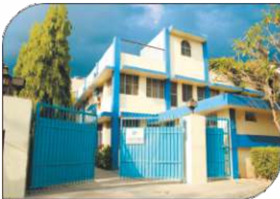
THE FACTORY AT GURGAON
