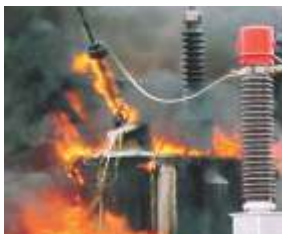
Moisture ingress into Bushing
